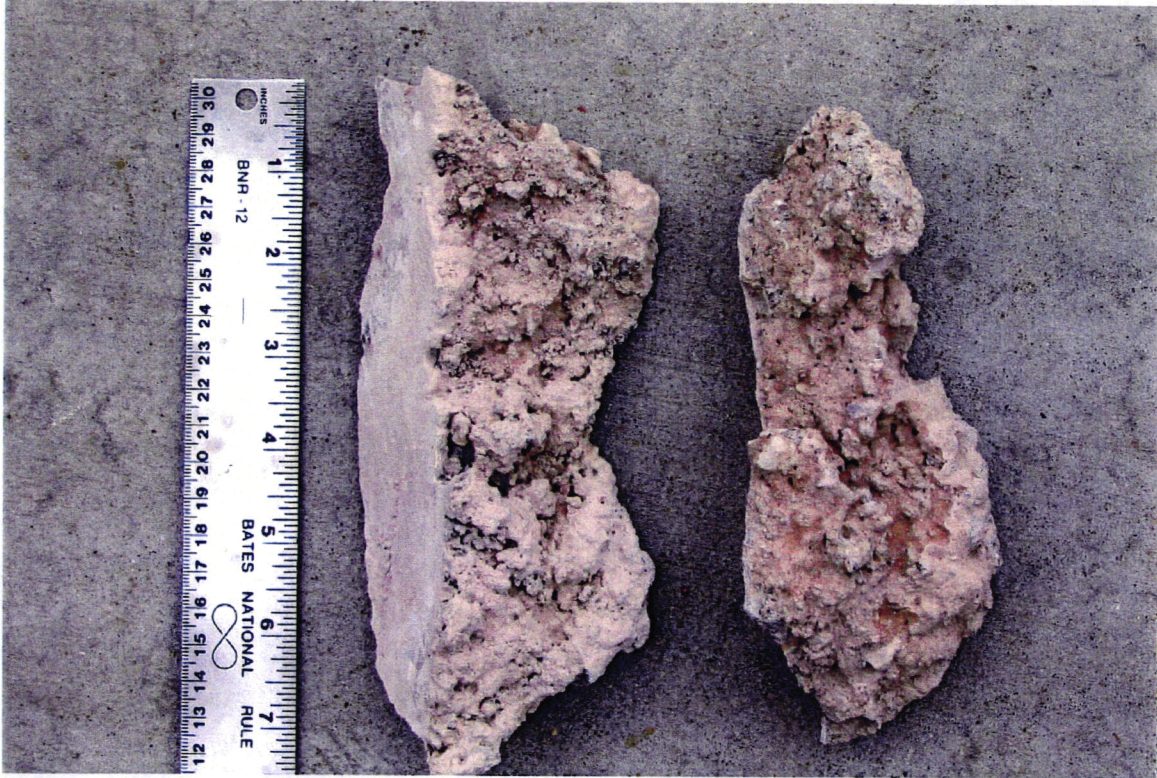
SAMPLE ID: P3 DESCRIPTION: Sawcut section of concrete as recieved.
