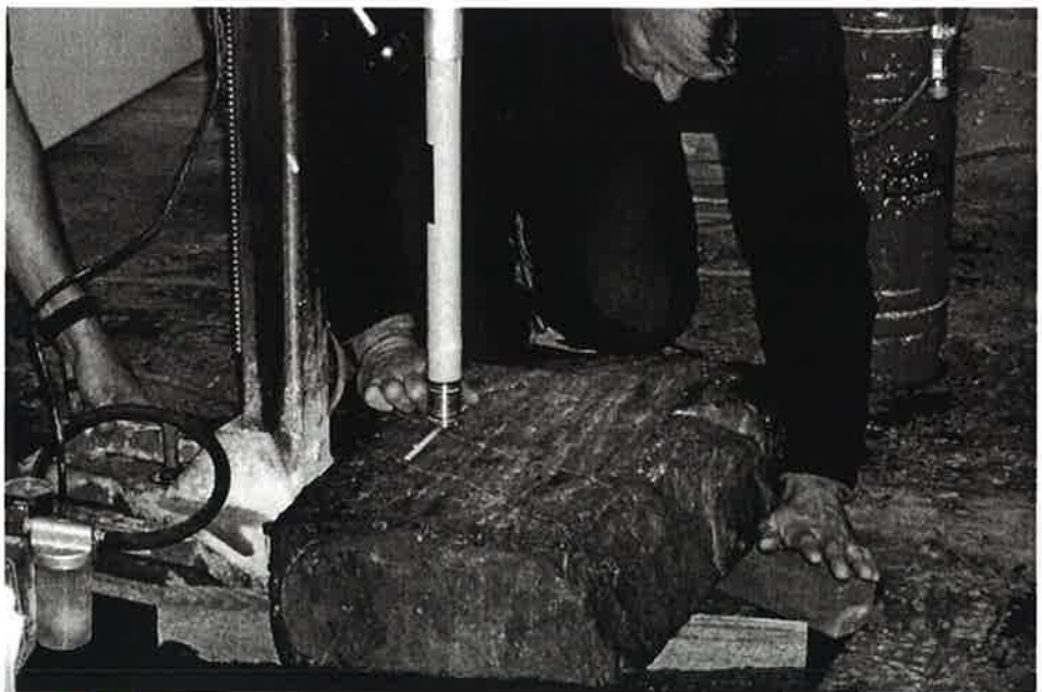
✓ The 1-1/4" (32 mm) diameter diamond-studded coring bit being positioned on October 3, 2000.
