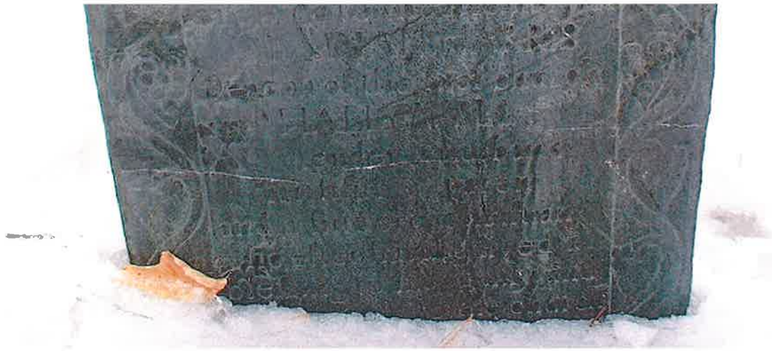
Figure #53: White-colored secondary deposits exuding from sub-horizontal fractures traversing the face of a slate tombstone.
