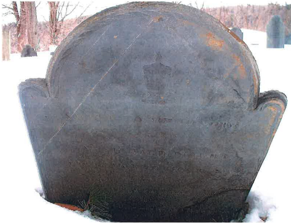
Figure #54: Sub-parallel fractures and rust-colored iron-oxide deposits on the face side of the Richard Dummer (1806) tombstone.
